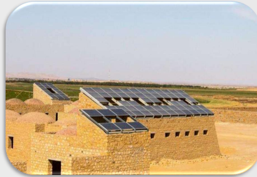
200kw Solar System Morocco year 2018
