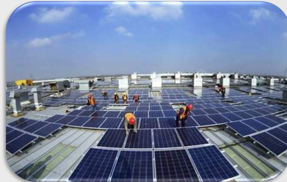
2MW Power Plant Portugal year 2018
