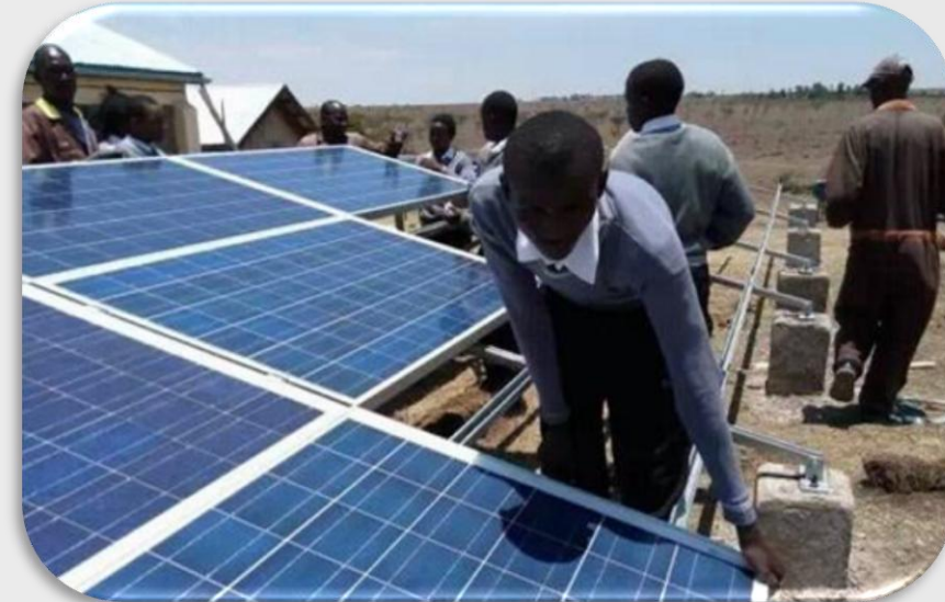
800kw Solar System Angola year 2018
