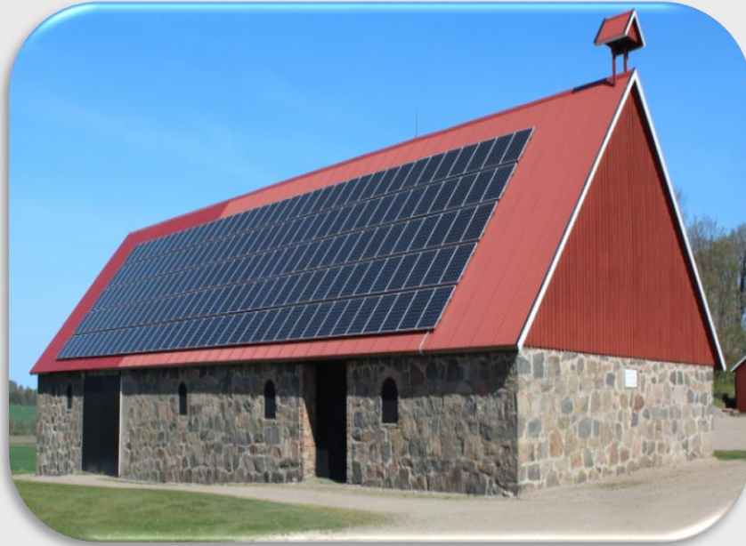
500KW Roof System Sweden year 2016
