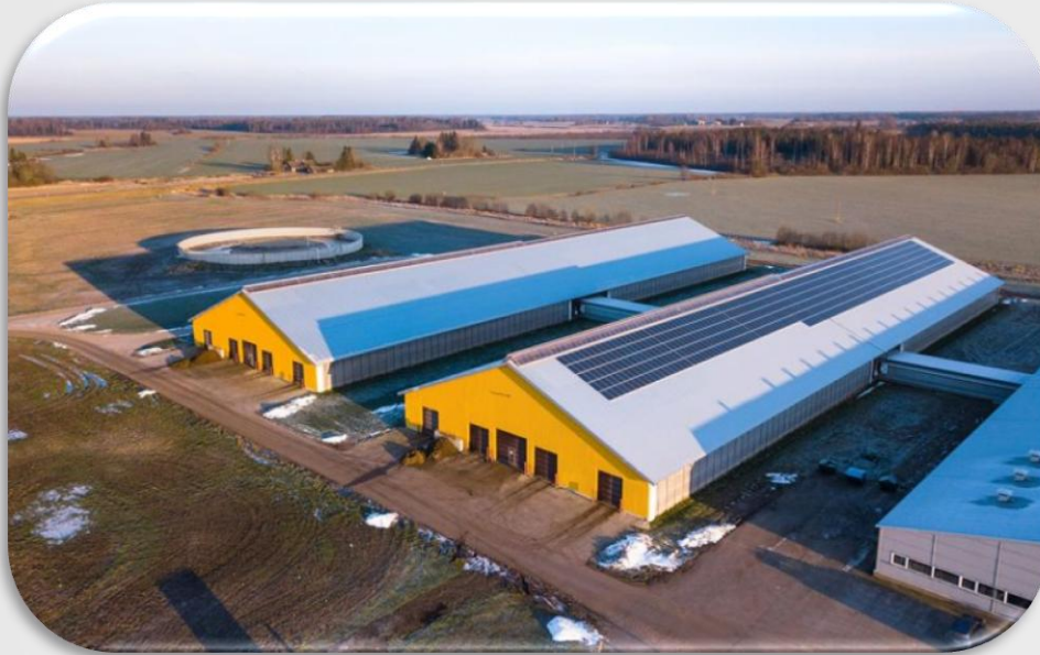
1.1MW Solar Power Plant Estonia year 2019
