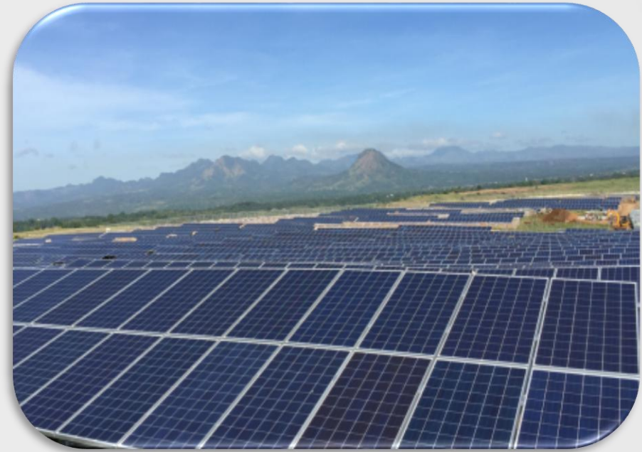
14.5MW Solar Power PV Station Philippines year 2015
