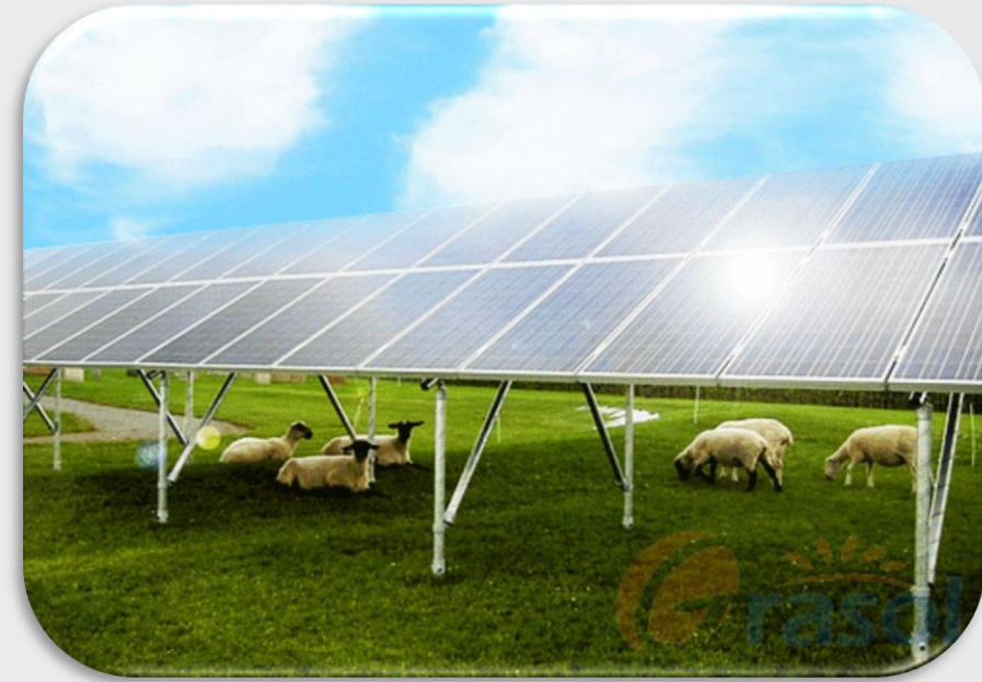
1MW Power Plant Switzerland year 2016
