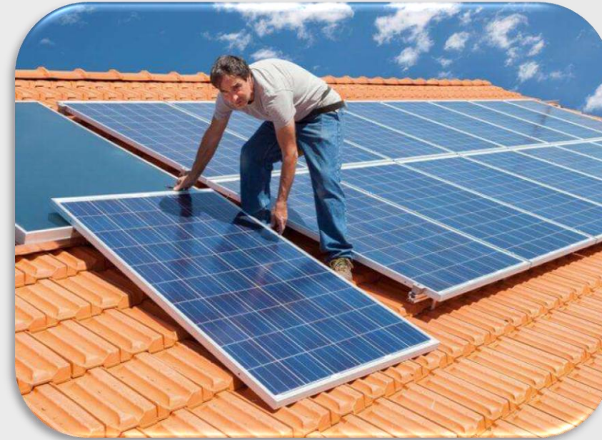
800kw Roof System Netherlands year 2014
