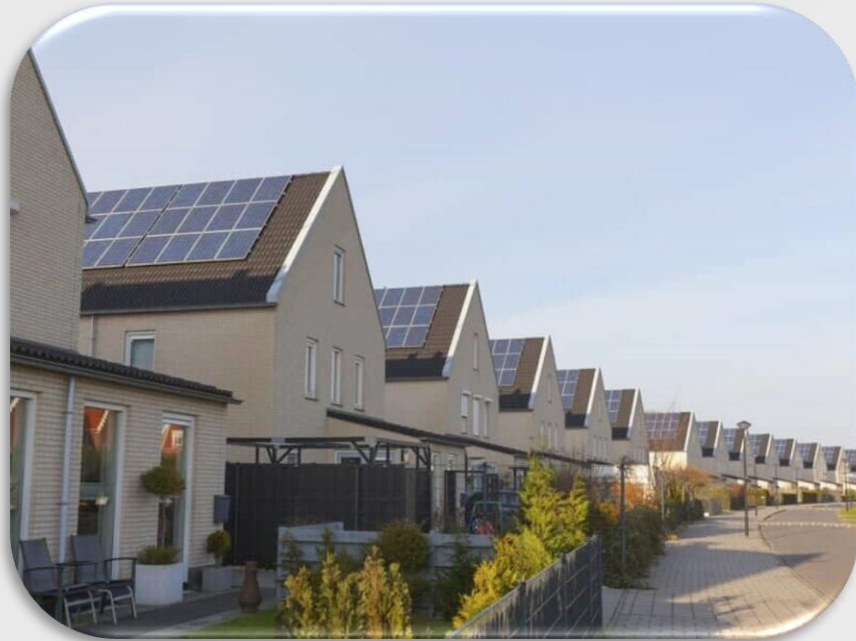
2MW Residential Roof System Germany year 2015
