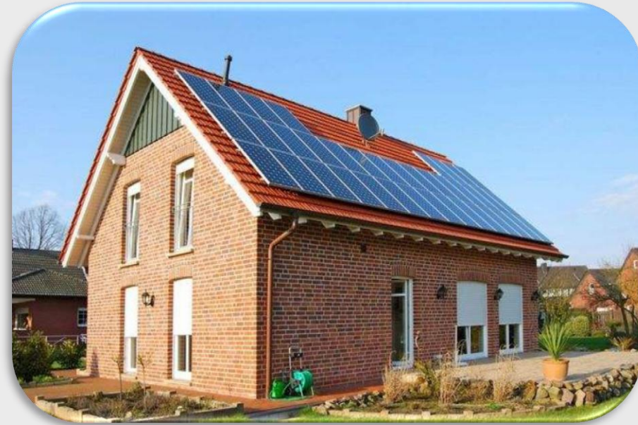
500kw Roof System Germany year 2014
