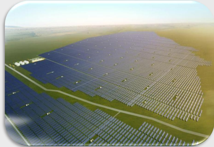
45MW Ground Solar Power PV Station Inner Mongolia , China year 2014
