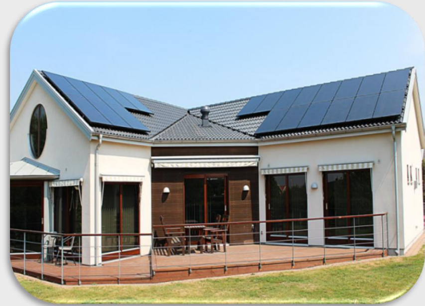
300KW Residential Roof Solar Power Sweden year 2016
